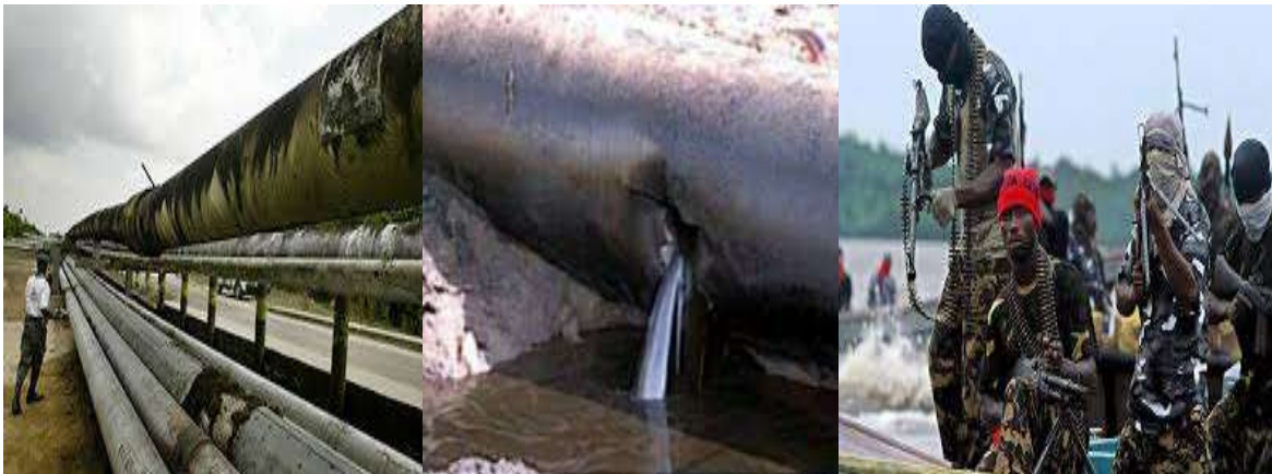
Pipeline Vandalization by militants
